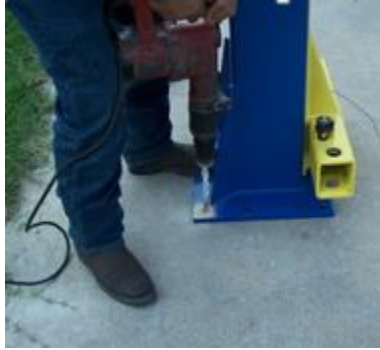
(Showing Installation of first Anchor Bolt)
